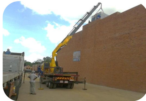
Hoisting of Aircon Units onto roof
