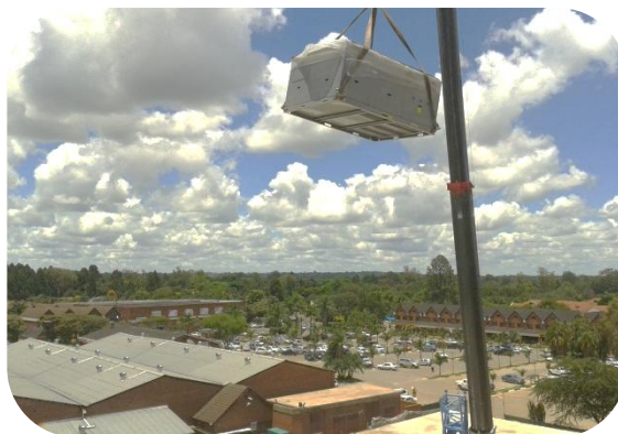
Hoisting of Aircon Units onto roof
